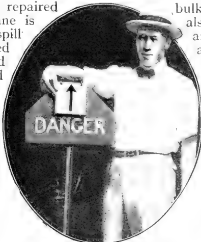
A heavy steel plate used to direct attention upward when the danger is from wires overhead
